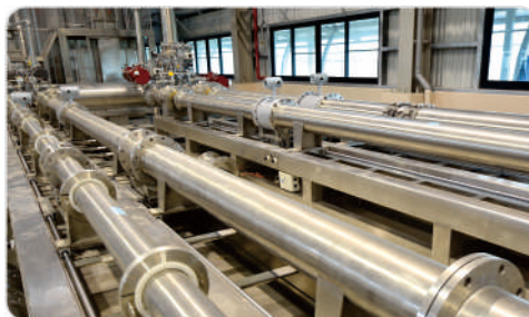
Piping system II (Maximum diameter is 500mm)
